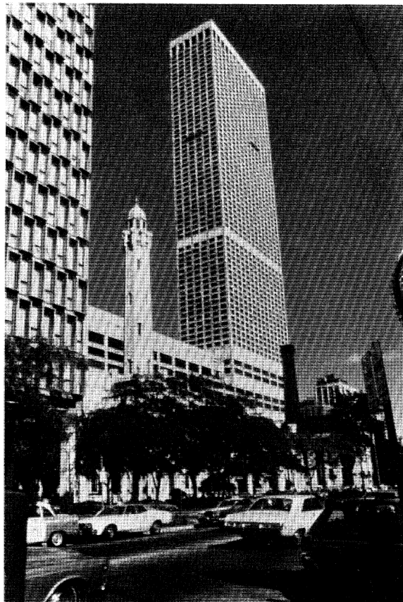
FIGURE 6. Improvements in cements and concretes can lead to improvements in civil engineering. The Water Tower Place in Chicago is the world’s tallest reinforced concrete frame building ( ca. 260 m). The structural columns of its lower floors were constructed with 62 MPa (90 days) ready-mixed concrete, which was not available until about 10 years ago.
