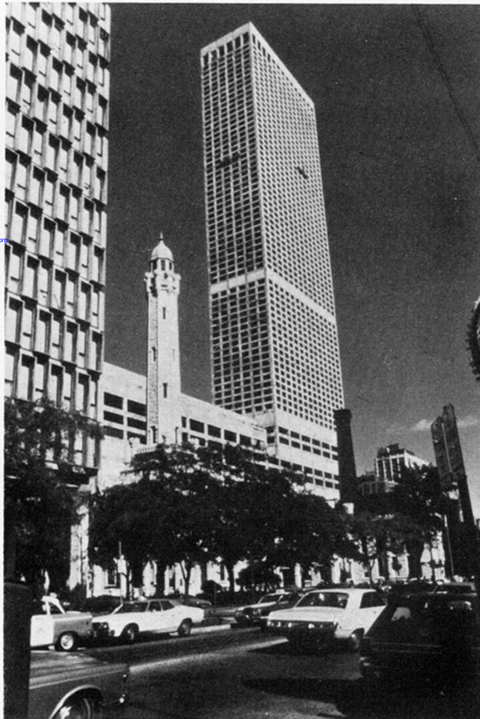
FIGURE 6. Improvements in cements and concretes can lead to improvements in civil engineering. The Water Tower Place in Chicago is the world's tallest reinforced concrete frame building ( ca. 260 m). The structural columns of its lower floors were constructed with 62 MPa (90 days) ready-mixed concrete, which was not available until about 10 years ago.
